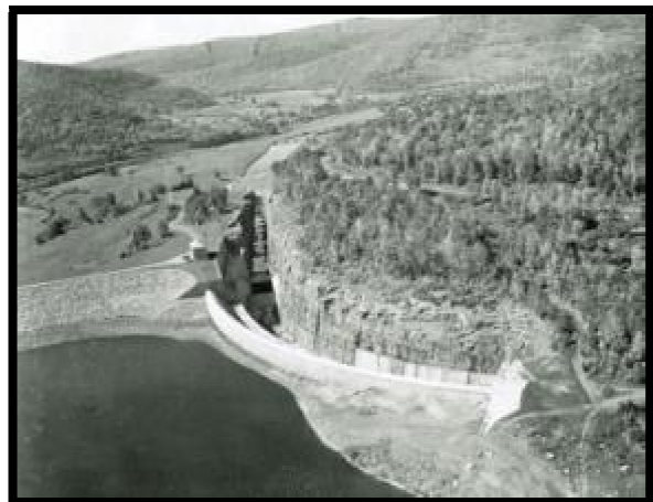
Aerial view of Dam and Spillway
